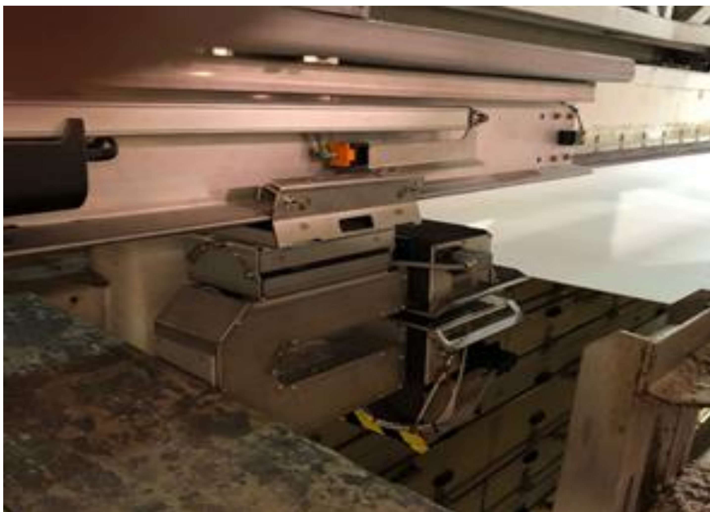
Fixed Point inverted C-frame installation
